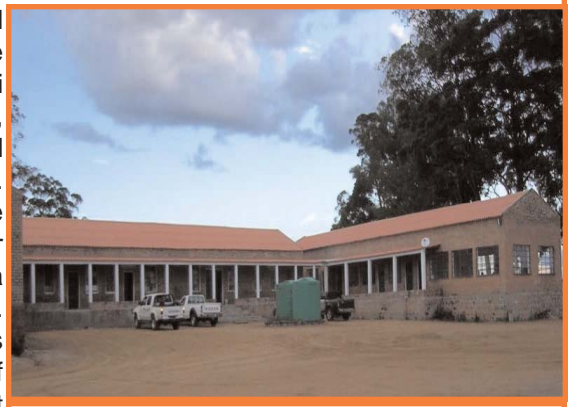
Dondi hospital, just reconstructed.
